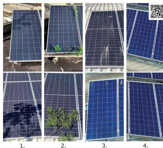
Fig. 2 Sample images of each class: 1 shadow class, 2 obstruction class, 3 dirty class, and 4 clear class. The QR Code contains the address to access the public dataset
