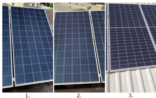
Fig. 5 Examples of images misclassified using MobileNetV3Large before fine-tuning. All these images were supposed to be classified as clear, but they were instead classified as follows: 1 obstruction, 2 shadow, and 3 dirty
