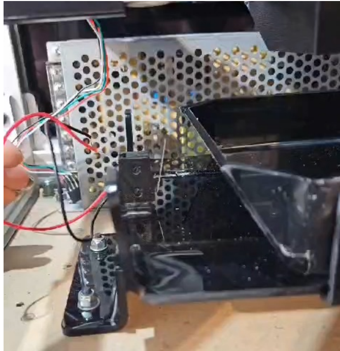
Figure 19: Limit Switch of Return Container
